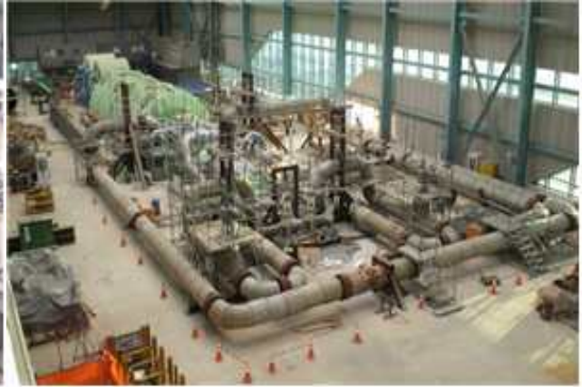
#2 증기터빈 Steam Blowing
