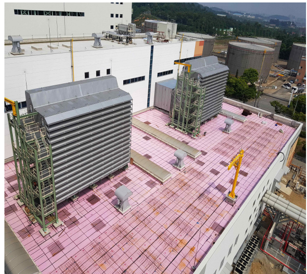
GT Low Roof
