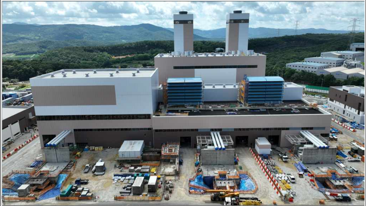
Power Block 전경
